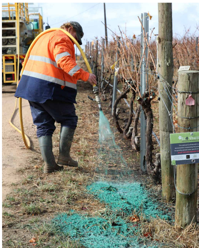
Figure 7: LCS Environmental hydroseeding equipment demonstration, autumn 2024 [Photo. Janet Klein].
