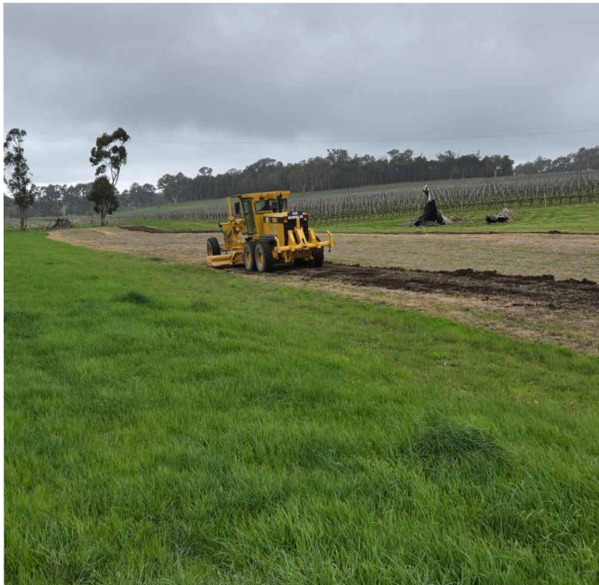
Figure 2: Soil preparation using a dozer to emulate the seed-burying moldboard plough action prior to seeding by Earthworks Tarra Civil [Photo: Simon Tolley].
