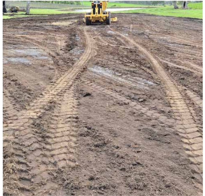
Figure 3: Soil preparation using a dozer to emulate the seed-burying moldboard plough action prior to seeding by Earthworks Tarra Civil [Photo: Simon Tolley].
