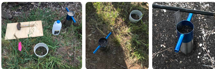
FIGURE 15: Installing a water infiltrator [Photos: Mary Retallack]
