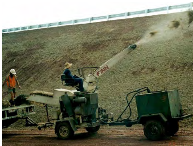
Figure 63. Hydroseeding (left), hydromulching (right) [Photos: Ian Chivers].
